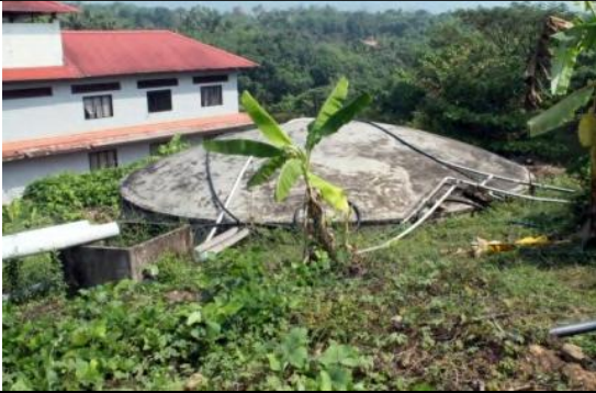
Rain Water Harvesting from Hostels - 15 lakh liters storage tank
