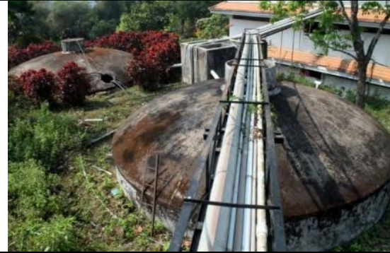
Rain Water Harvesting from Hostels - 15 lakh liters storage tank
