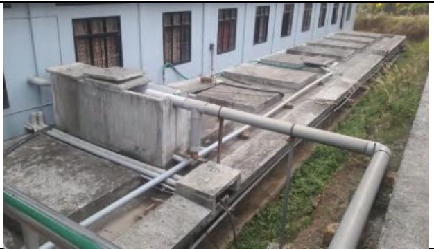
Rain Water Harvesting from Lecture blocks-26 lakh liter capacity, storage tanks at the rear side of the building
