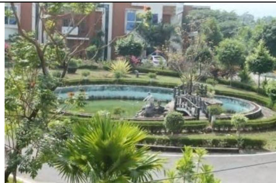
Rain Water Harvesting - 2 lakh liters capacity
