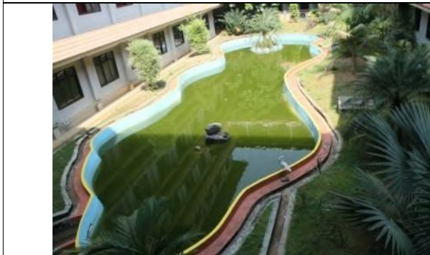
Rain Water Harvesting - 4 lakh liters capacity
