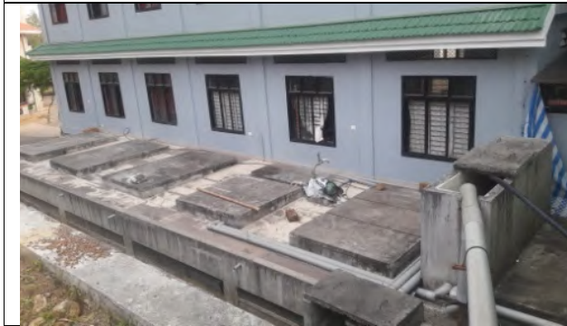
Rain Water Harvesting from Lecture blocks-26 lakh liter capacity, storage tanks at the rear side of the building
