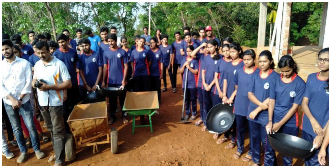
Renovation of GUPS school cheriya arikkamala (December 22nd and 23rd, 2018)
