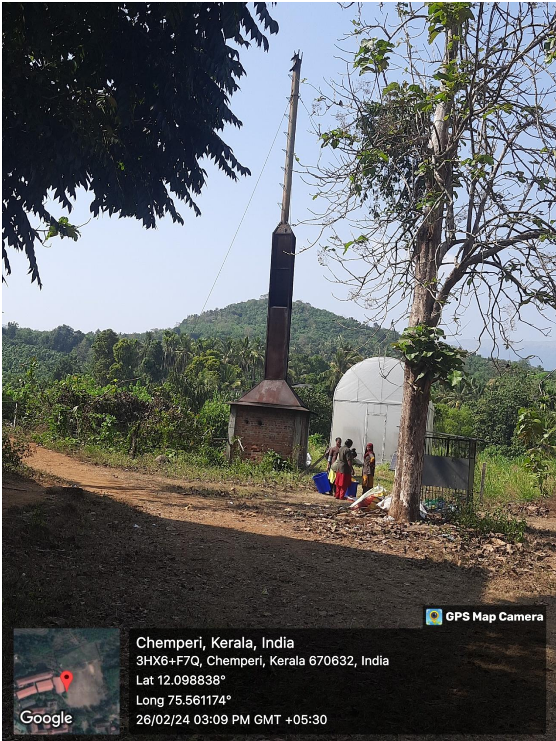
Incinerator in the campus getting ready for operation
