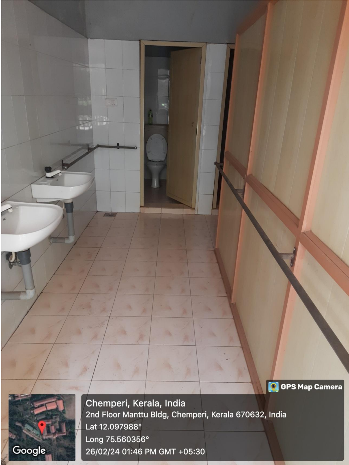
Close view of the hand rails inside the toilet
