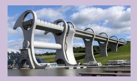
Completed in 2002, the Falkirk Wheel is the world's first and only rotating boat lift. It was designed to connect the Forth and Clyde Canal with the Union Canal.
