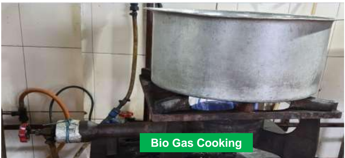
Bio Gas Stove and units
