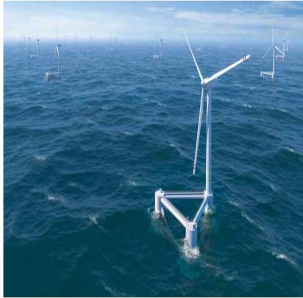
Fig. 3.2 WindFloat turbine with semi-submersible floater (source: www.ewea.org )
