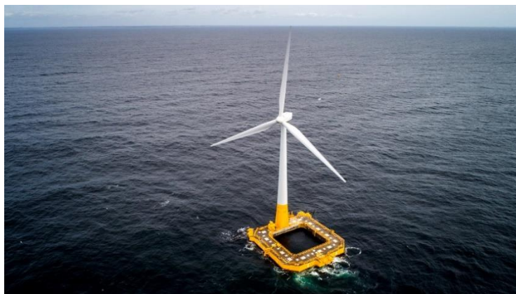
Fig. 1.6 IDEOL'S offshore wind turbine
