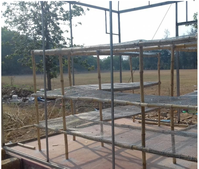
Figure 4: Bamboo rack installation
