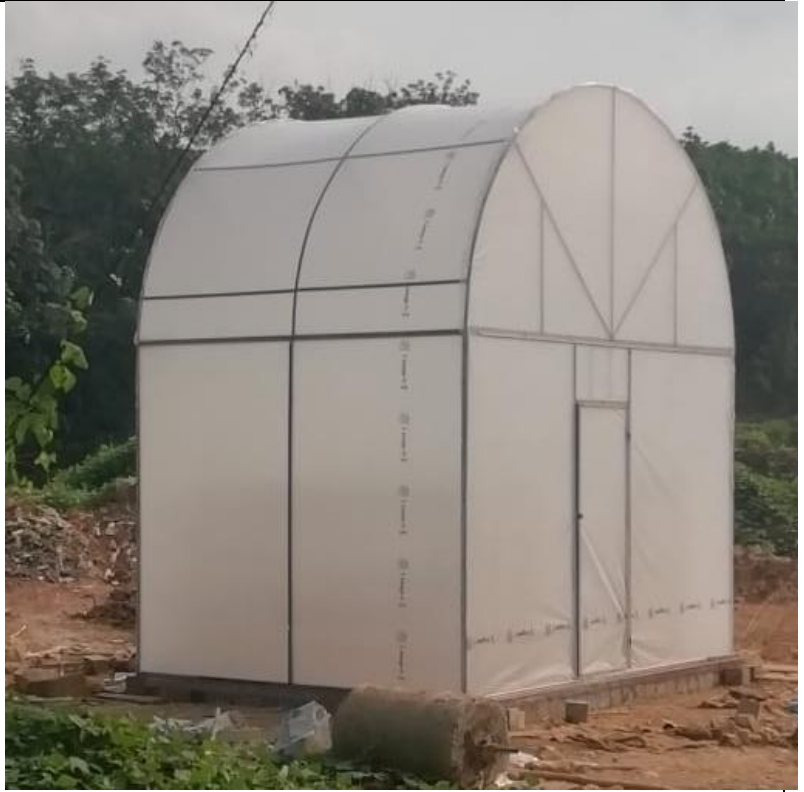
Figure 5: Installation of UV stabilized film
