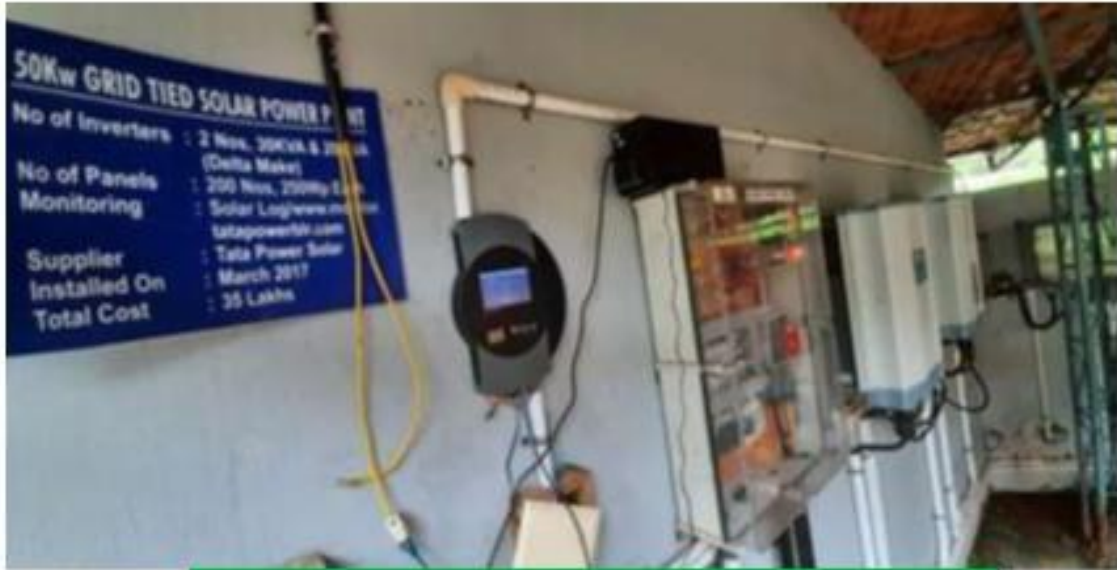
50 kW Solar panel connected to the KSEB Grid
