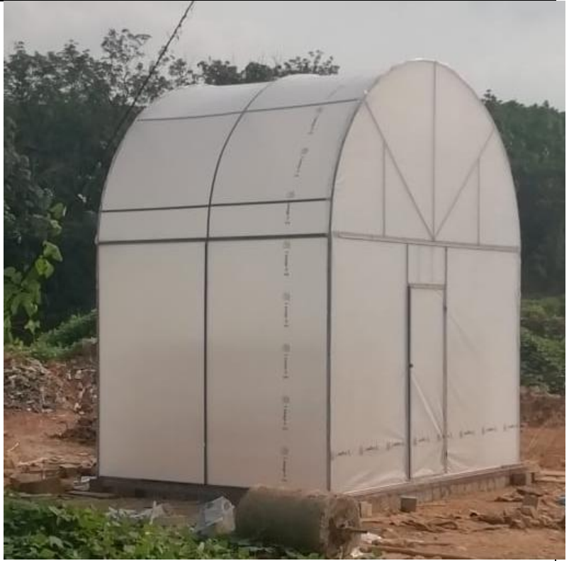
Figure 5: Installation of UV stabilized film
