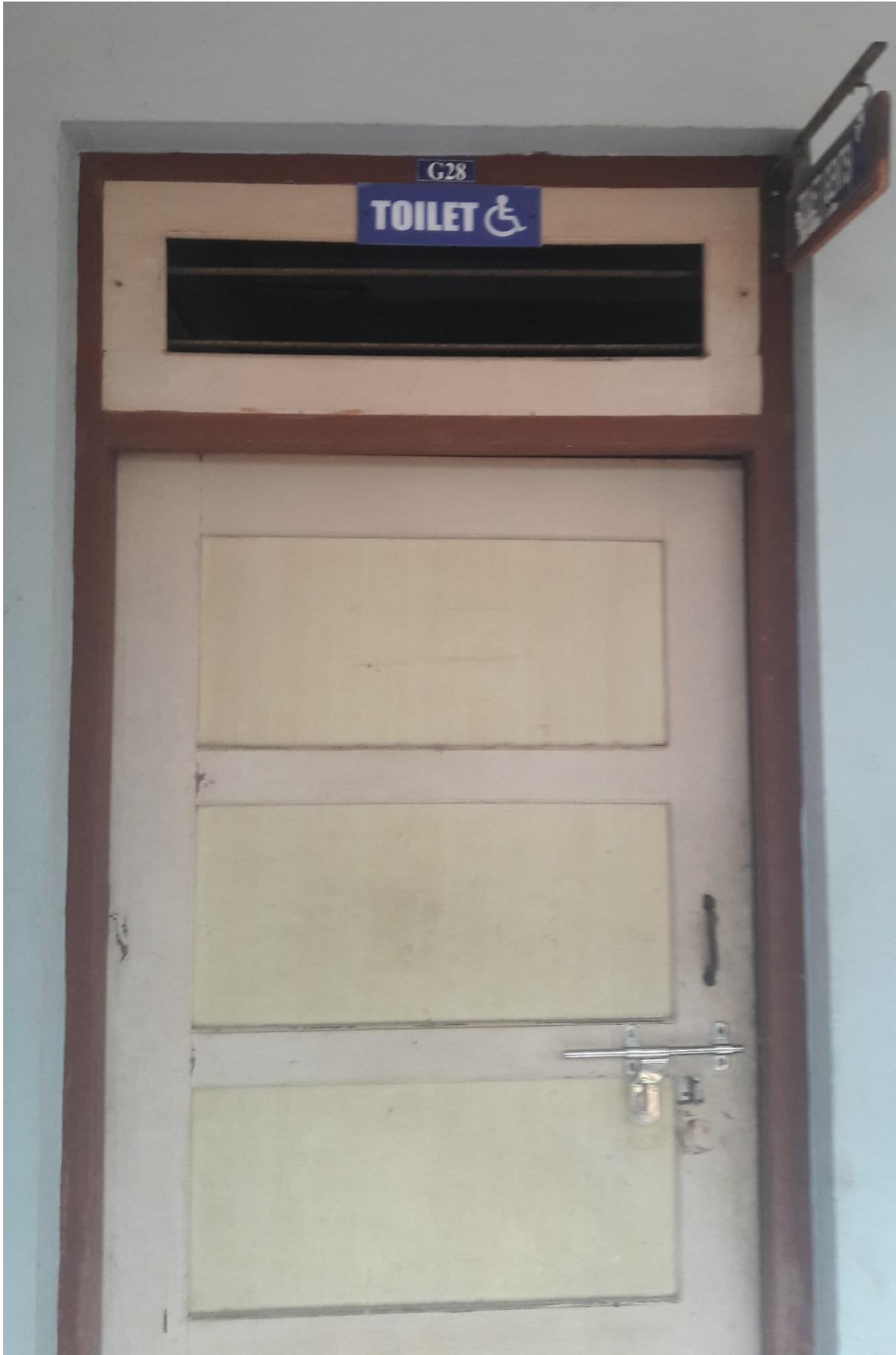
Toilet for specially talented (handicap) people
