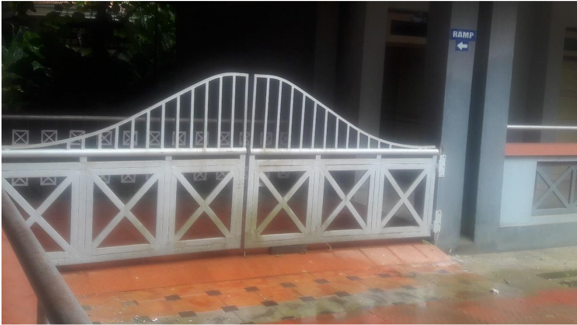
Ramp provided for specially talented (handicap) people to enter the college
